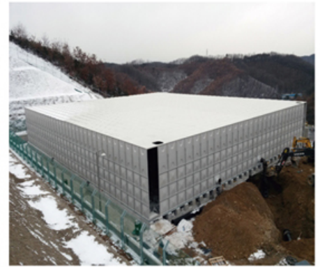
Roof Panel assembly
