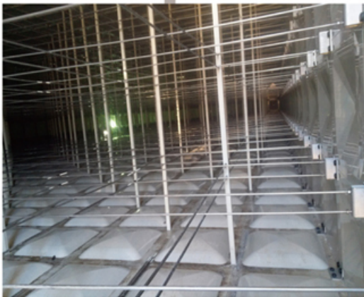
Internal tie-rod & Roof support assembly
